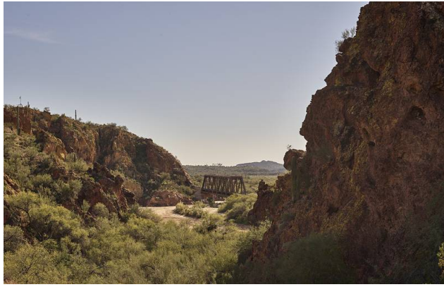
Fig. 99. Railroad bridge in a canyon outside Wickenburg (2018-11-16) Highsmith, Carol M., 1946-, photographer; No known restrictions on publication (LOC; Carol M. Highsmith Archive, donated to public domain) · source
