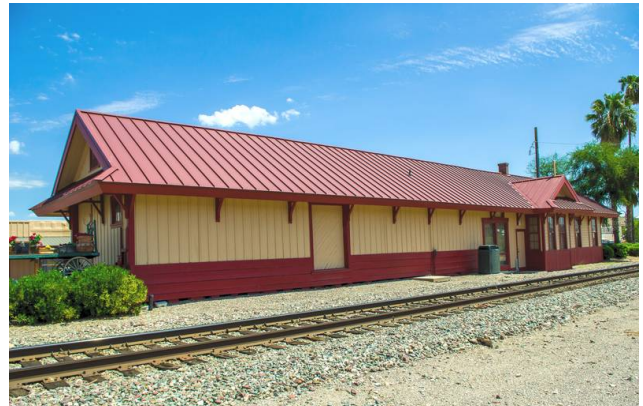
Fig. 86. Former Santa Fe station in Wickenburg, Arizona. Built in 1895 by Santa Fe, Prescott & Phoenix Railway. Now used as a museum and city offices. (Replaces a photo originally posted in March 2007.) (2017-08-23) Ron Reiring; CC BY 2.0 (per Wikimedia Commons) · source
