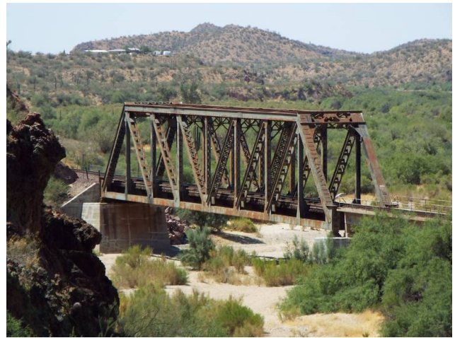
Fig. 84. Pratt through truss BNSF Railroad Bridge, built in 1930, across the Hassayampa River in Wickenburg, Az. (2017-07-02) Marine 69-71; CC BY-SA 4.0 (per Wikimedia Commons) · source
