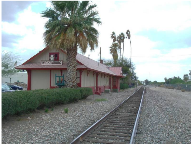
Fig. 63. Santa Fe Railroad Depot — built 1875, and located at 215 N. Frontier in Wickenburg, Arizona. The property was listed in the National Register of Historic Places in July 10, 1986. Reference number #86001588 (2013-04-09)
