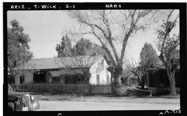
Fig. 26. South Flont [Frontier] Street (House), Wickenburg, Maricopa County, AZ (HABS AZ-54) (1940) Delos H. Smith, photographer (Historic American Buildings Survey); No known restrictions on images made by the U.S. Government (HABS); images copied from other sources may be restricted · source
