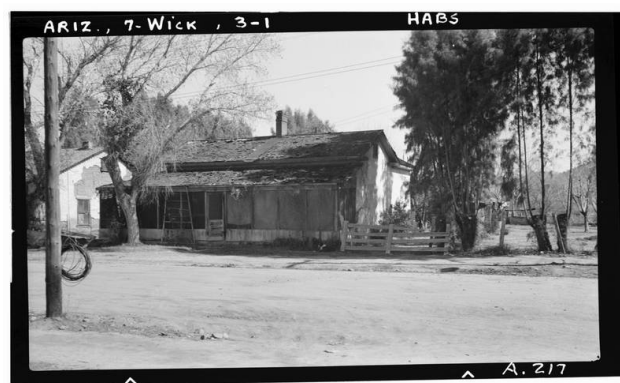
Fig. 29. South Flont [Frontier] Street (House), Wickenburg, Maricopa County, AZ (HABS AZ-53) (c1940 (HABS; companion record az0045 photographed 1940 by Delos H. Smith)) Historic American Buildings Survey; No known restrictions on images made by the U.S. Government (HABS); images copied from other sources may be restricted · source
