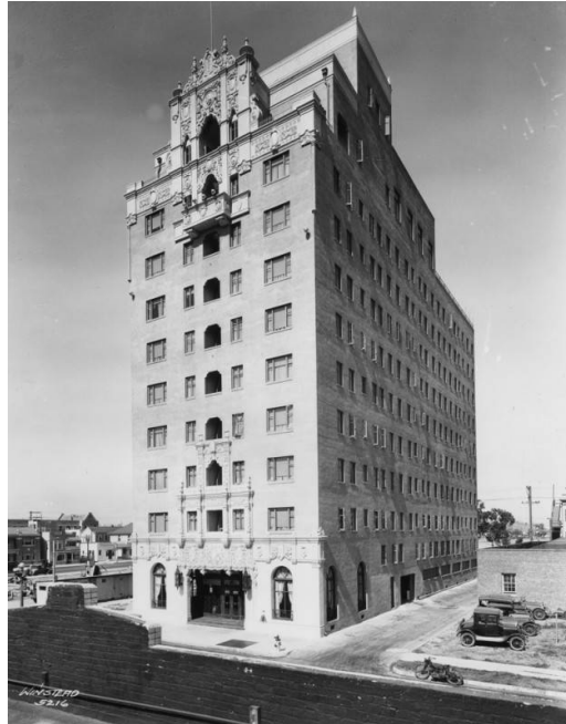
Fig. 1 Campbell Apartments, 130 Linden Avenue, 1928 (Winstead Photo).
